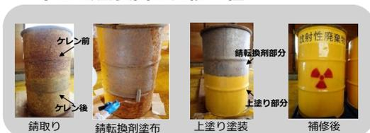
Fig.1 Drum cans storing low-level radioactive waste.
